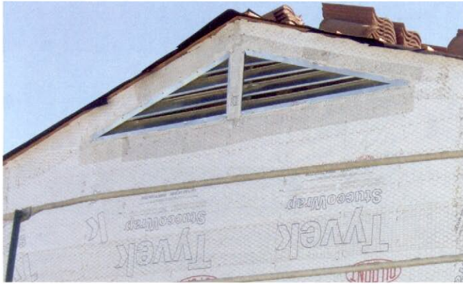
Tyvek stucco wrap at the doors, walls and windows act as a barrier to manage moisture and control airflow.
